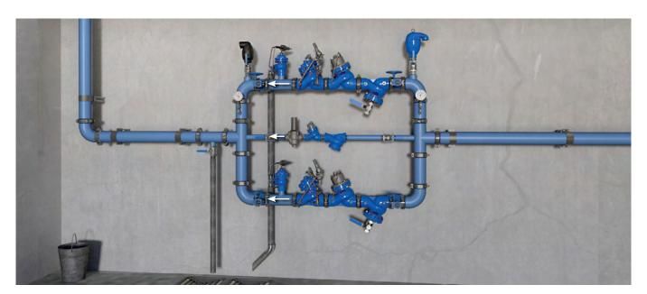
Pressure Reducing Station, featuring BERMAD BC-80F-P Strainers to protect each branch from foreign debris, a redundant, parallel branch to minimize the possibility of total water shut-off and a low flow bypass branch for low demand operation. For information on the other BERMAD products in this system please see the product data sheet for the following components: BERMAD BC-820-PD-P, BERMAD BC-720-P and BERMAD BC-73Q-P.
